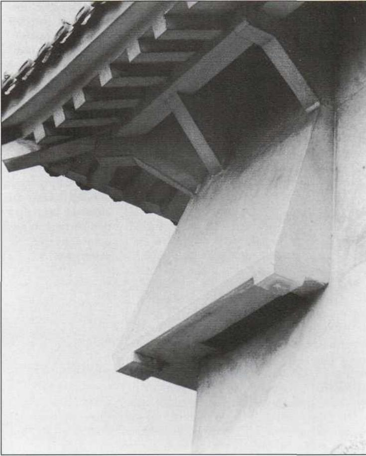
**Above:** A loophole at Himeji, for dropping rocks down on to attackers, or for firing guns and bows.
